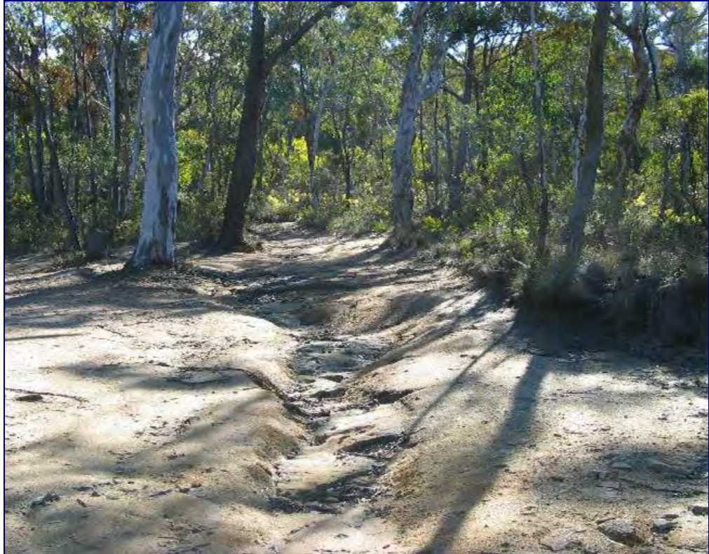
Figure 15: Another example of heavily eroded, overused vehicle tracks.
