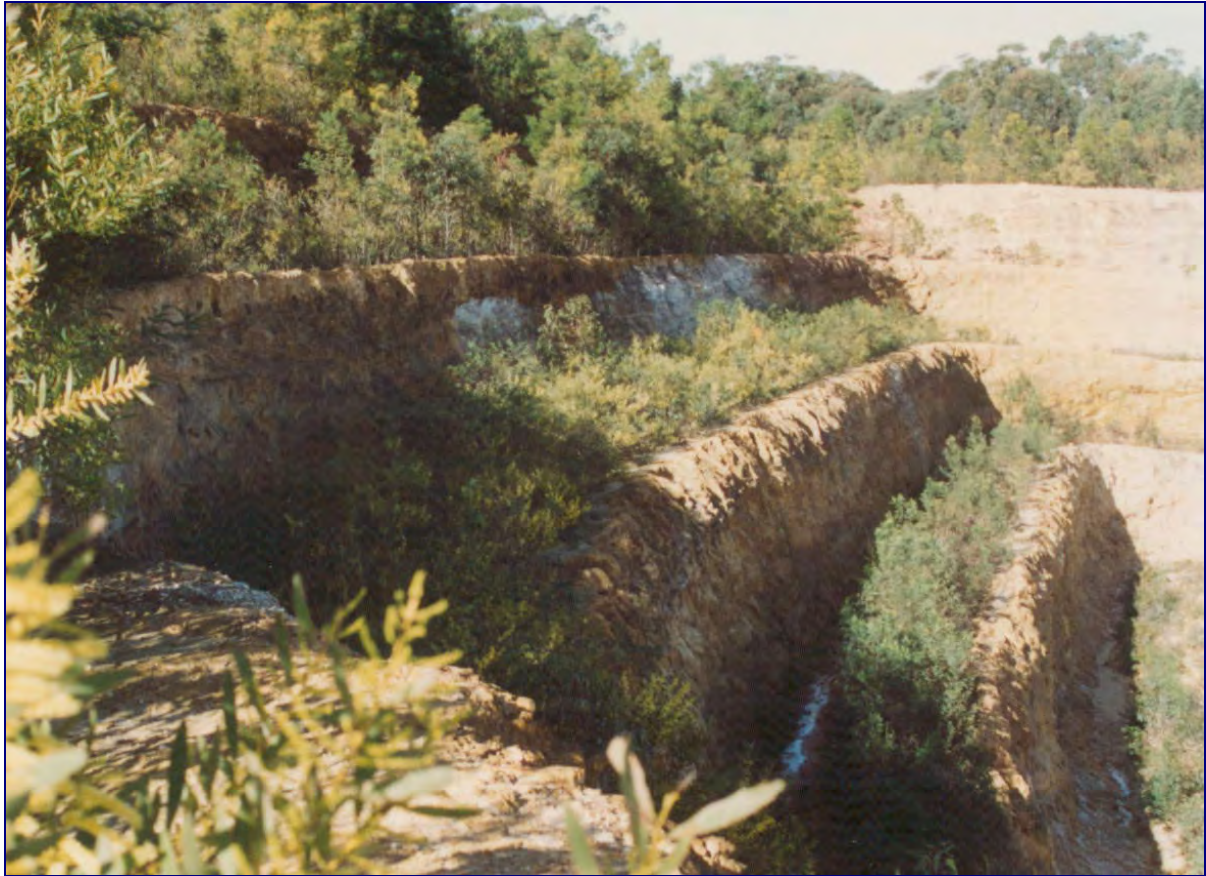
Figure 3: Progressive rehabilitation – top bench: 3 yrs old, bottom bench: 6 mon. old.
