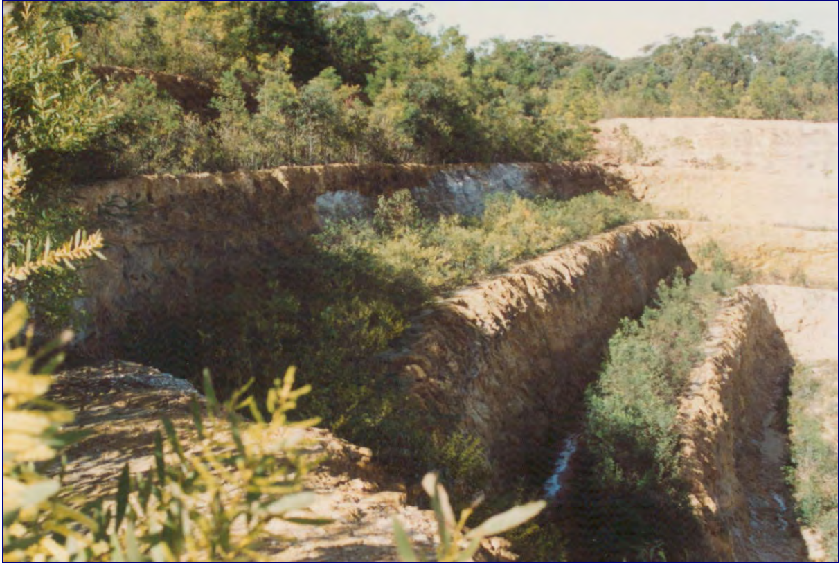
Figure 14: Progressive rehabilitation – top bench: 3 yrs old, bottom bench: 6 months old (Mark Burns, Global Soil Systems)
