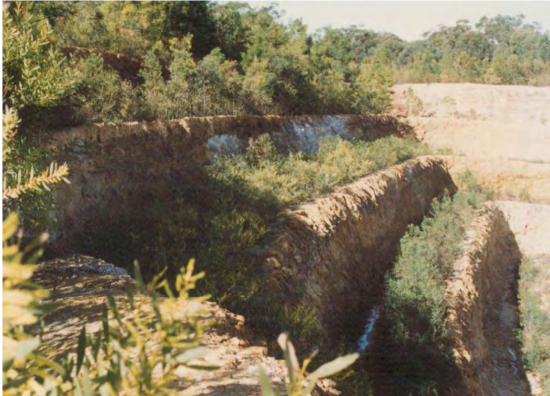
Figure 9 - Actual terraced landscaping in progress
